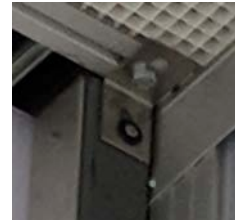
ceiling attachment with 2"x2" L-bracket
